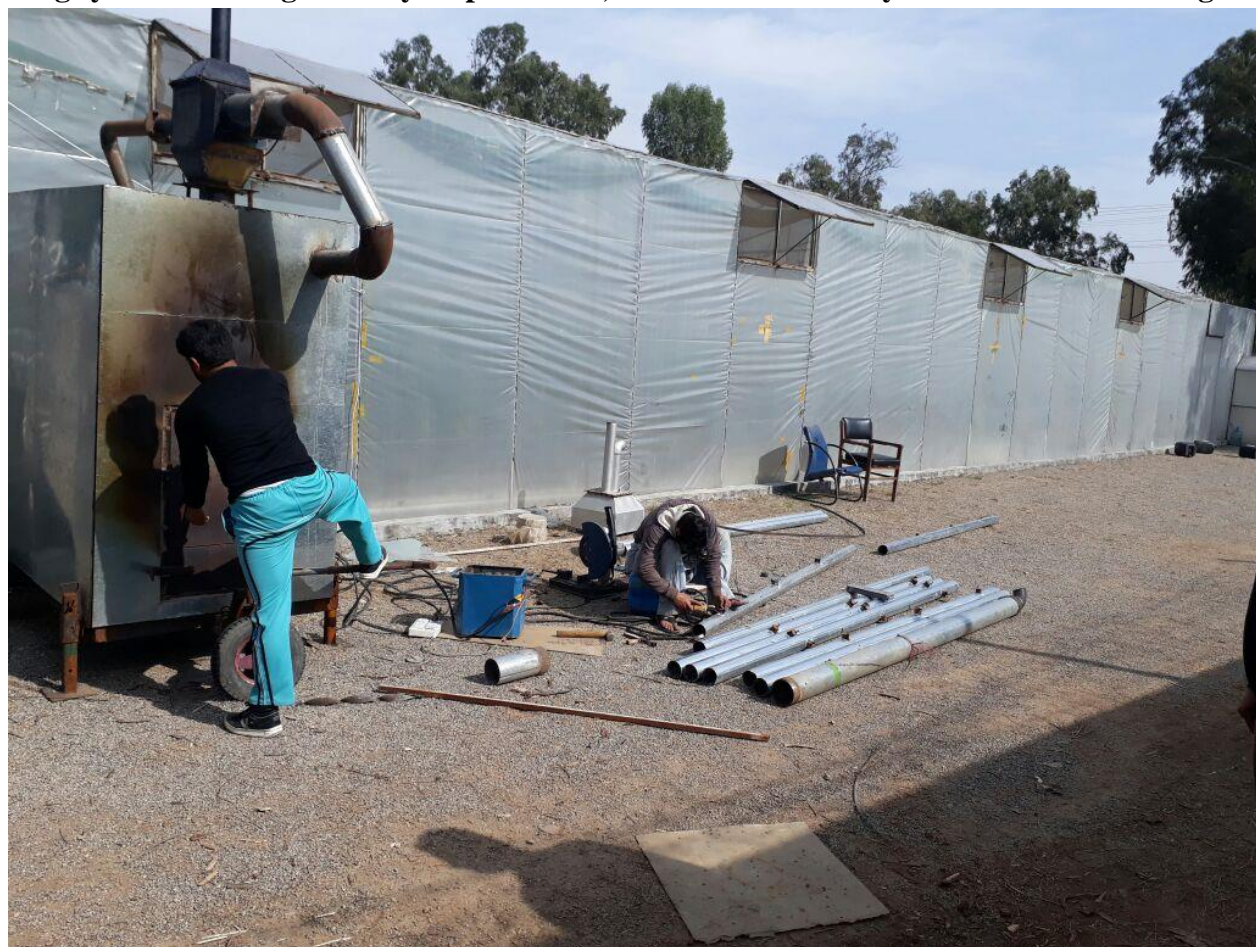
Heating system for indigenous hydroponic unit, it uses the university solid waste for heating the unit.
