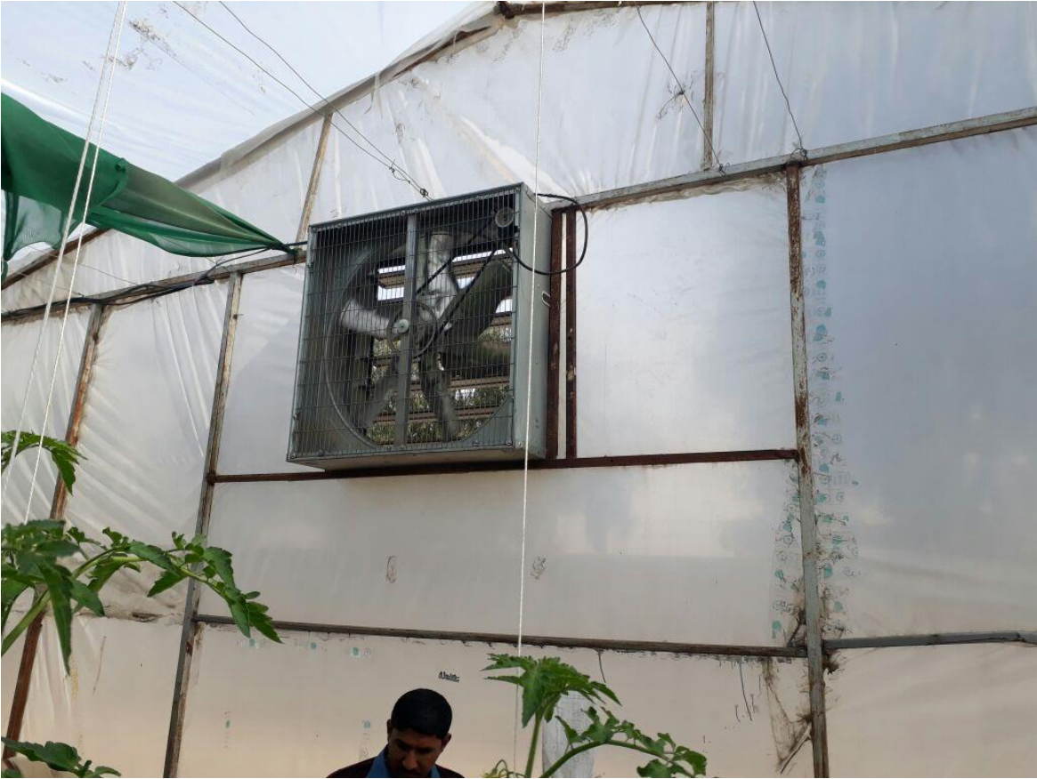
Ventilation system in indigenous hydroponic unit
